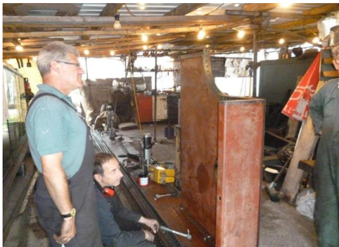
Dave and Martin working on the cab end of one of the tanks in the early stages of assembly in 2013. The 'bunko-booth' has now changed out of all recognition.
