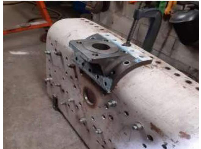
Well done Dick - it fits! We never doubted your abilities. The new mounting pad trial fitted to the back head, ready to be riveted. The steam take-off can be seen at the top.
